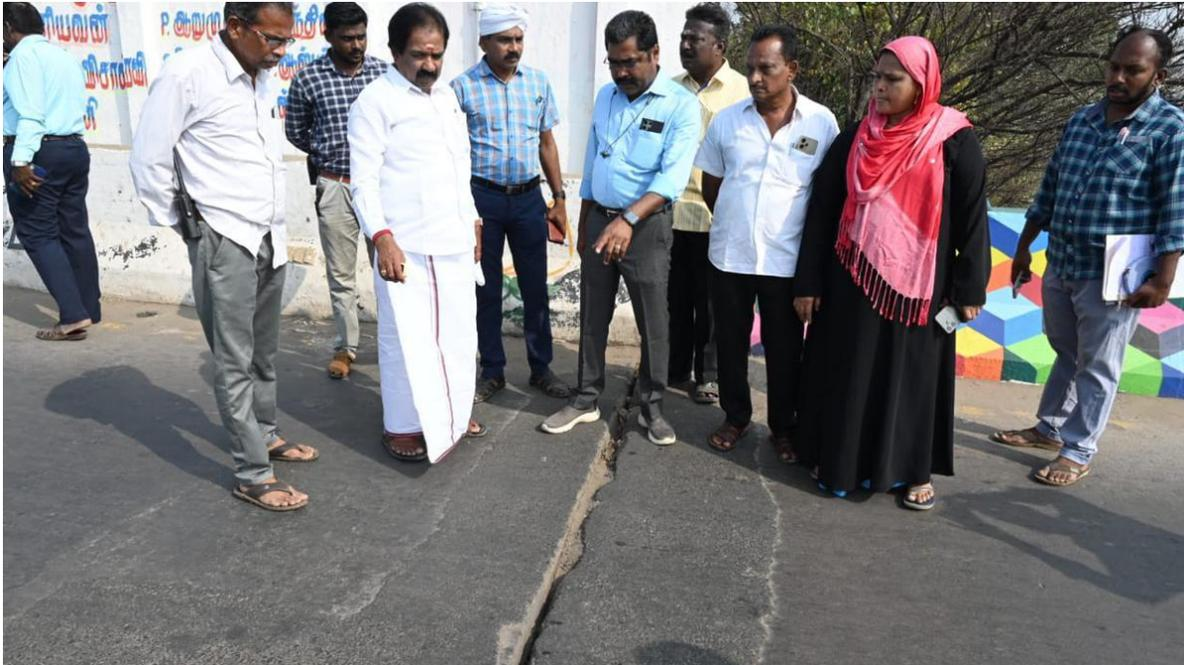
**Despite periodic repairs, it is a bumpy ride on the two overbridges because of widening gaps and damages to the expansion joints, say regular users of the road**
