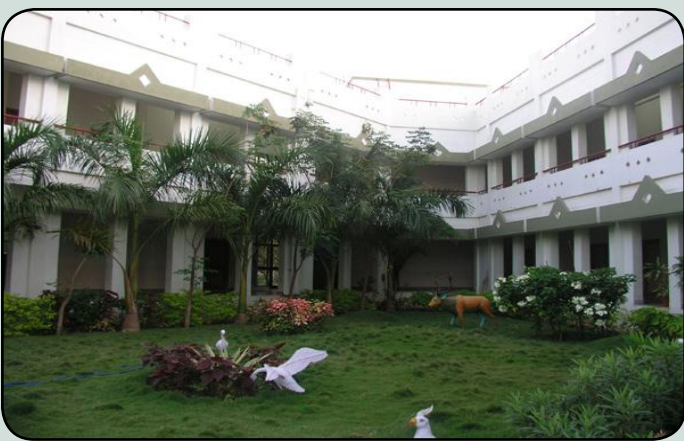
Lecture Hall Complex
