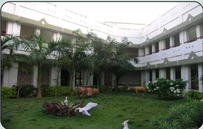
Lecture Hall Complex
